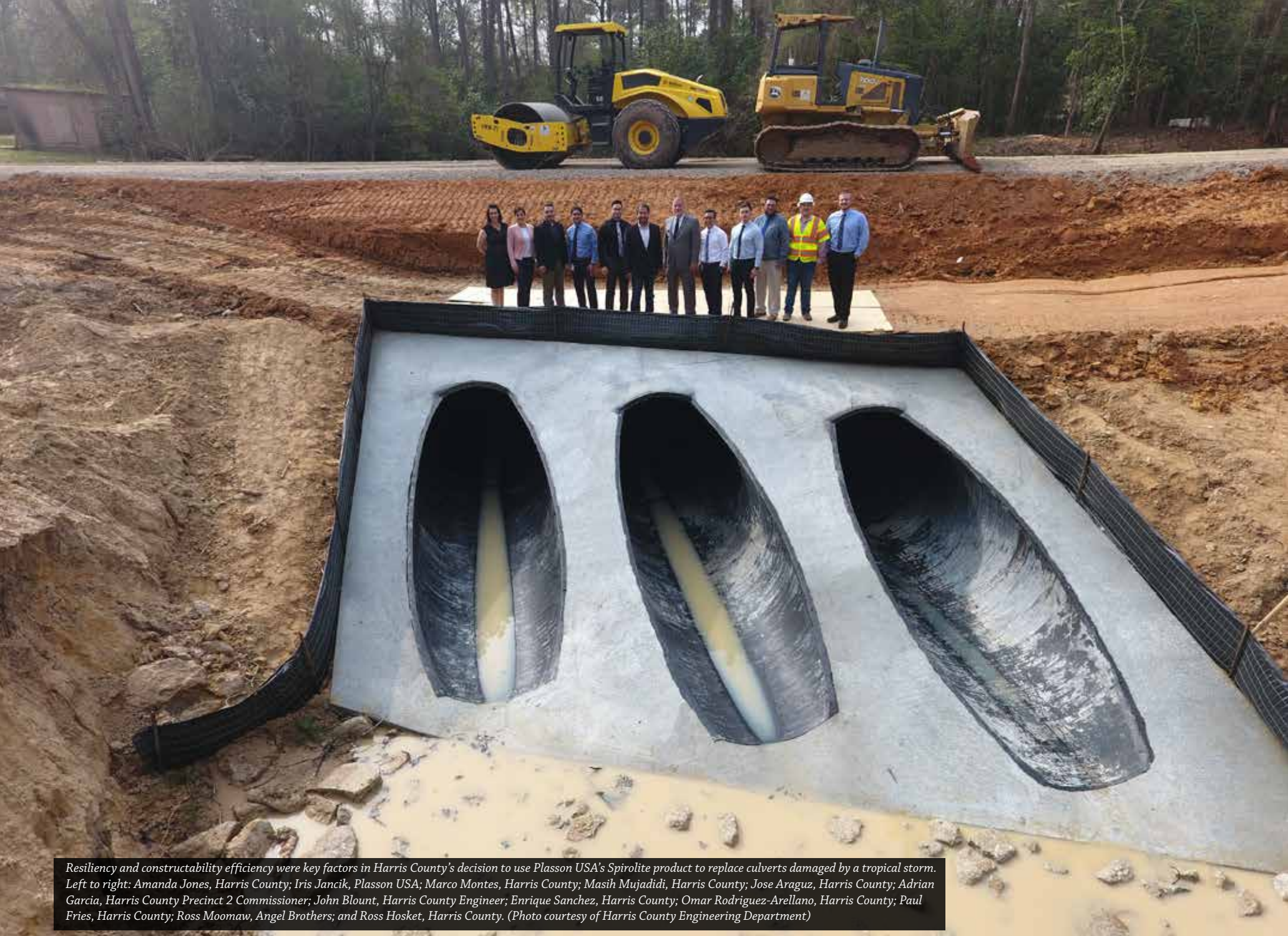
Spirolite, a specialized HDPE fluid network conveyance system, is a go-to solution for highway improvements nationwide. (Photo courtesy of Plasson USA)
